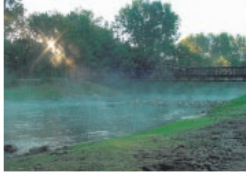
The new Mill Pond Dam area.
