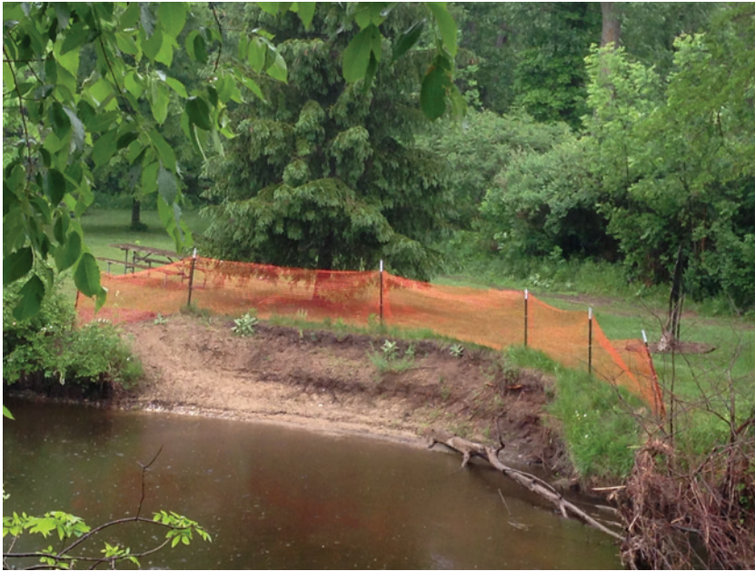
Erosion Near Swinging Bridge in 2014
